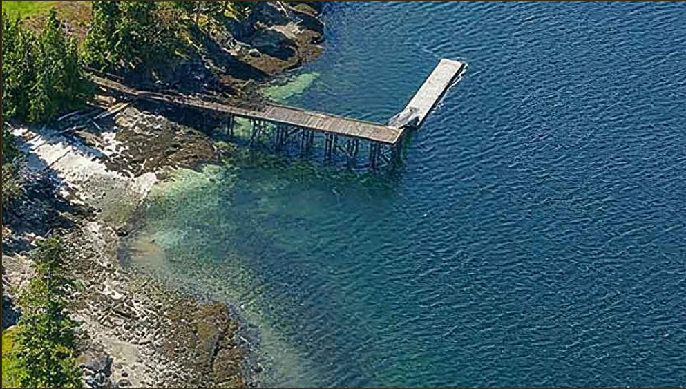
The pier and deep-water dock
