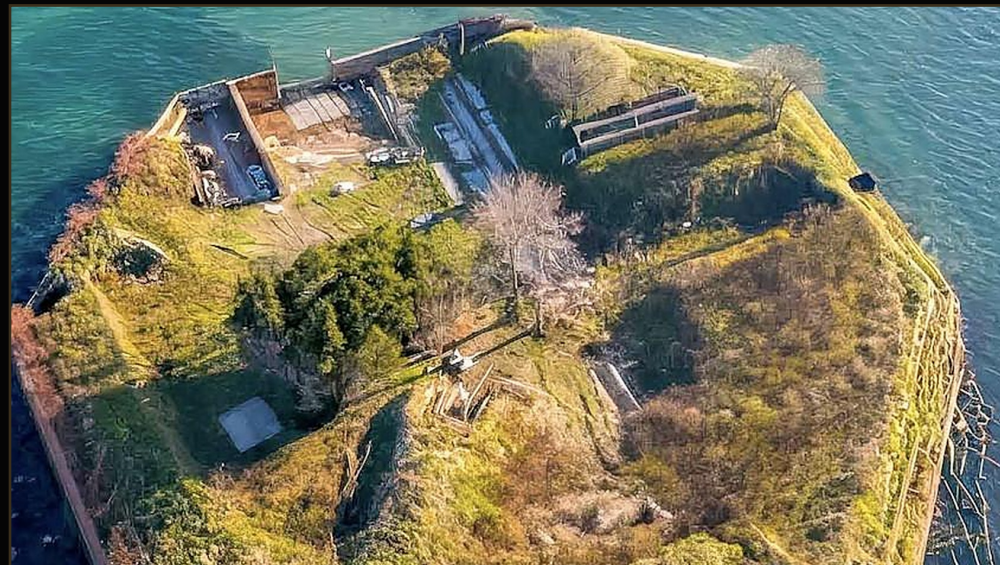
Earthworks and remains within the perimeter
