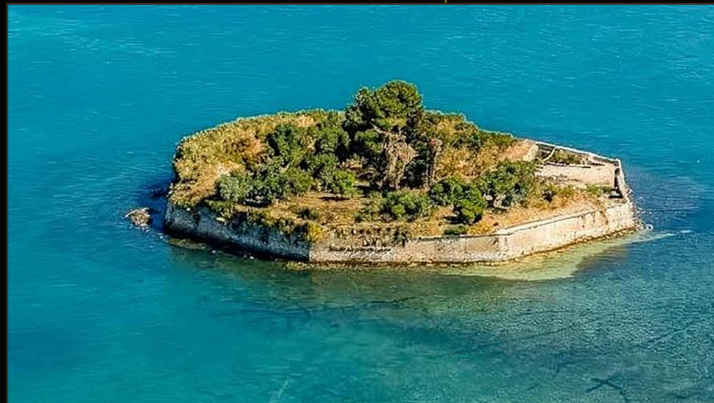
The stone perimeter from the water
