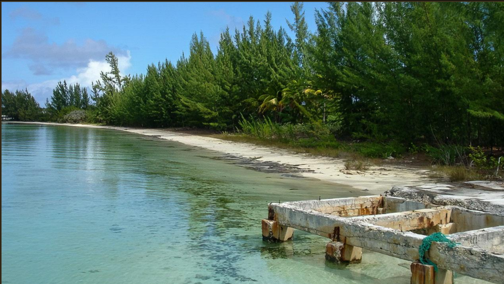
The former dock's foundation
