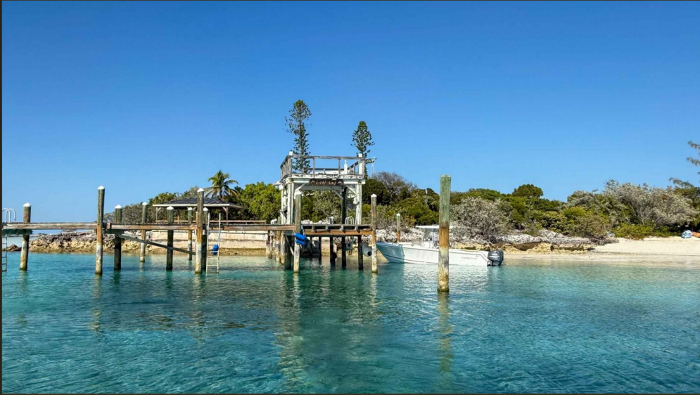
The dock from the anchorage
