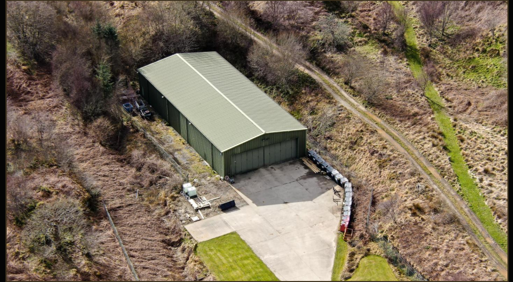
The helicopter hangar and apron
