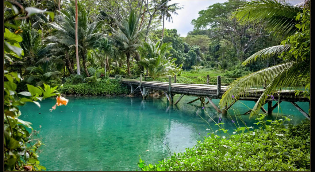
The footbridge over the inlet
